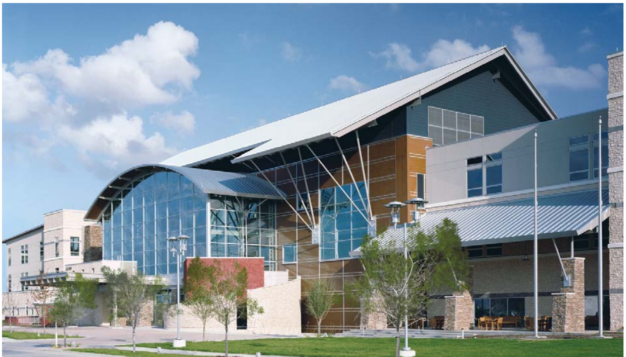
DESIGNED WITH HOSPITALITY IN MIND, CENTENNIAL MEDICAL CENTER IN FRISCO, TEXAS, LOOKS MORE LIKE A TEXAS HILL COUNTRY LODGE THAN LIKE A TYPICAL HOSPITAL. PHOTO CREDIT: © 2005 GARY KNIGHT + ASSOCIATES
