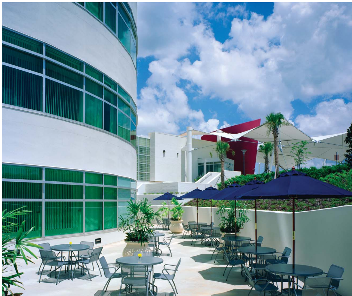
OUTDOOR DINING IS A HOSPITALITY-STYLE AMENITY AT FLORIDA HOSPITAL WATERMAN IN TAVARES, FLA. THE LARGE RED CONE IN THE BACKGROUND IS A WAYFINDING ICON THAT CLEARLY IDENTIFIES THE EMERGENCY DEPARTMENT ENTRANCE. PHOTO CREDIT: © 2005 GARY KNIGHT + ASSOCIATES
